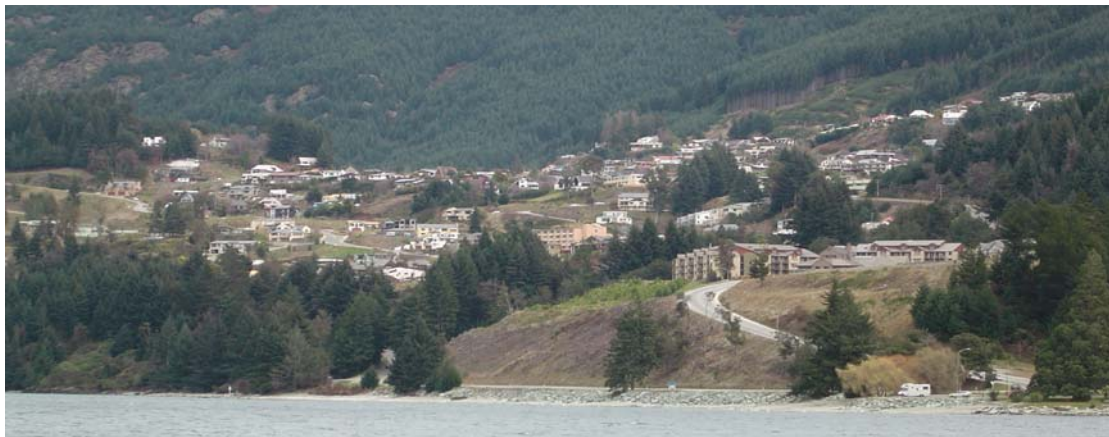
Figure 2 – Increasing low density development can detract from the value and appeal of the unique natural environment that gives Queenstown its character.
